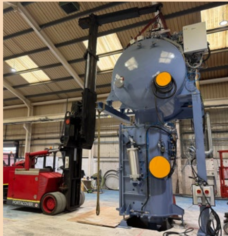
Vacuum Precision Investment Caster being installed at Wall Colmonoy's Pontardawe site
