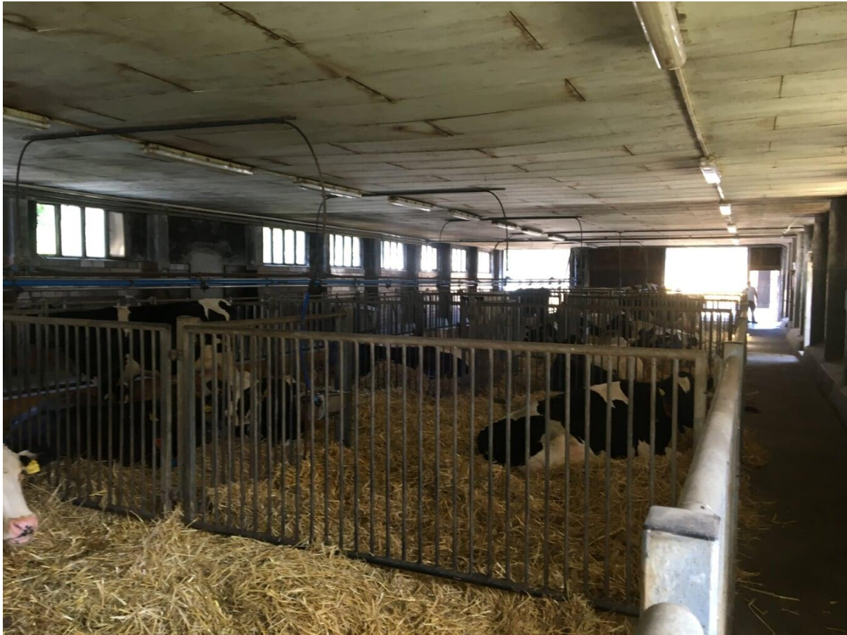
Fig 37. The older cow shed now used as calving pens/sick pens on loose housing, a vacuum line is in the building to allow the milking of any cows on antibiotics or freshly calved cows using a dump bucket
