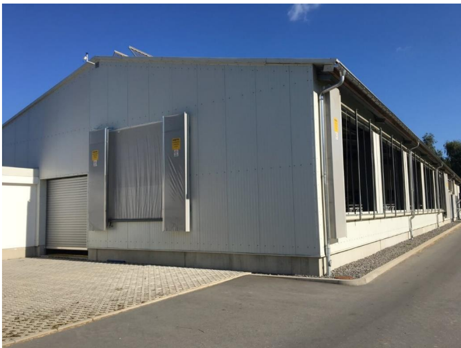
Fig 26. Shed housing collecting yard and robotic rotary parlour
