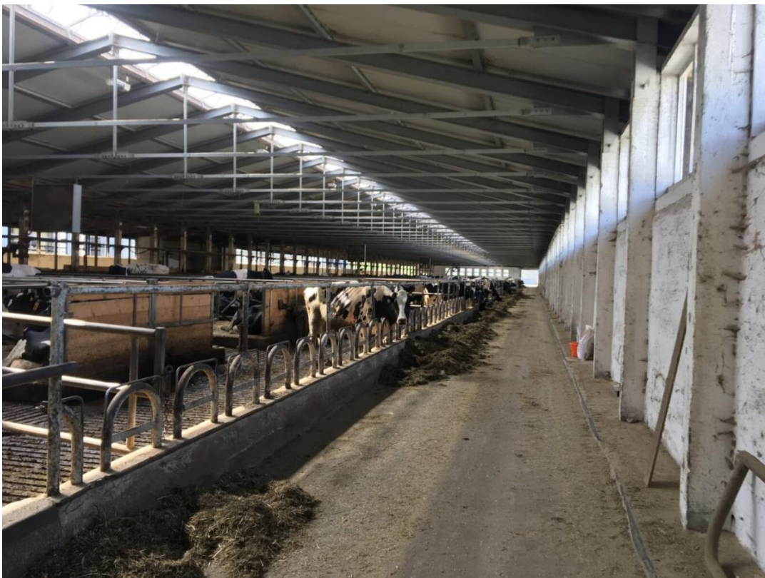
Fig 34. Bright and airy shed with the ridge of the roof opening and closing automatically
