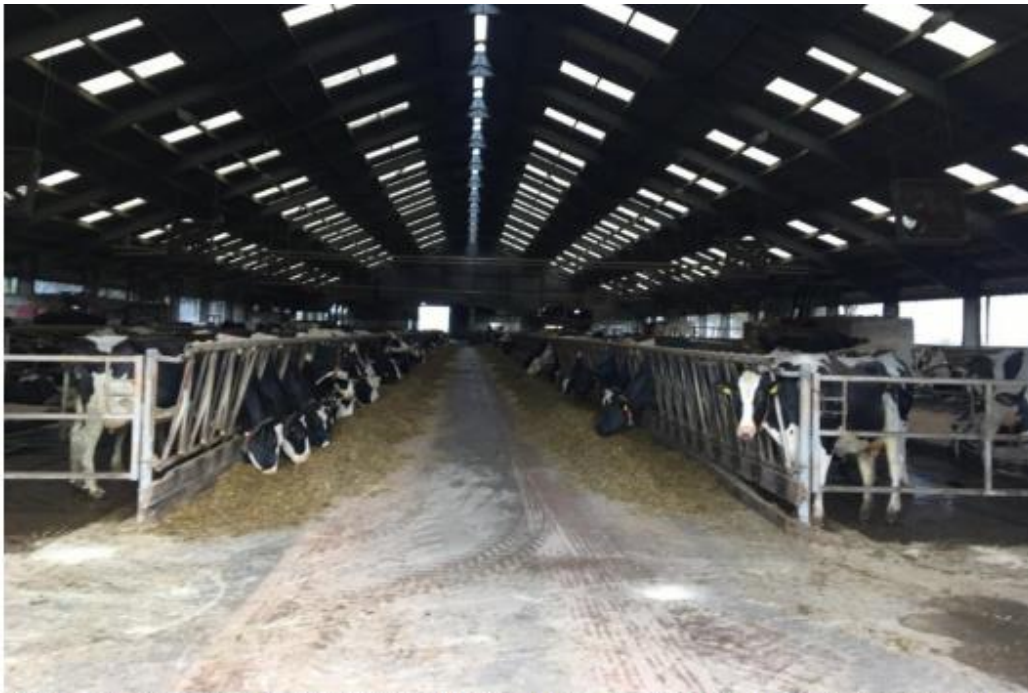
Main cattle shed housing the 6 Lely Astronaut Robots, high open peak on the roof to allow cool air to flow in through the open sides and the hot air to flow out through the roof.
