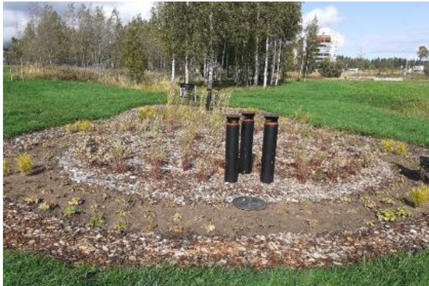
Fig 13. Underground biochar filter
