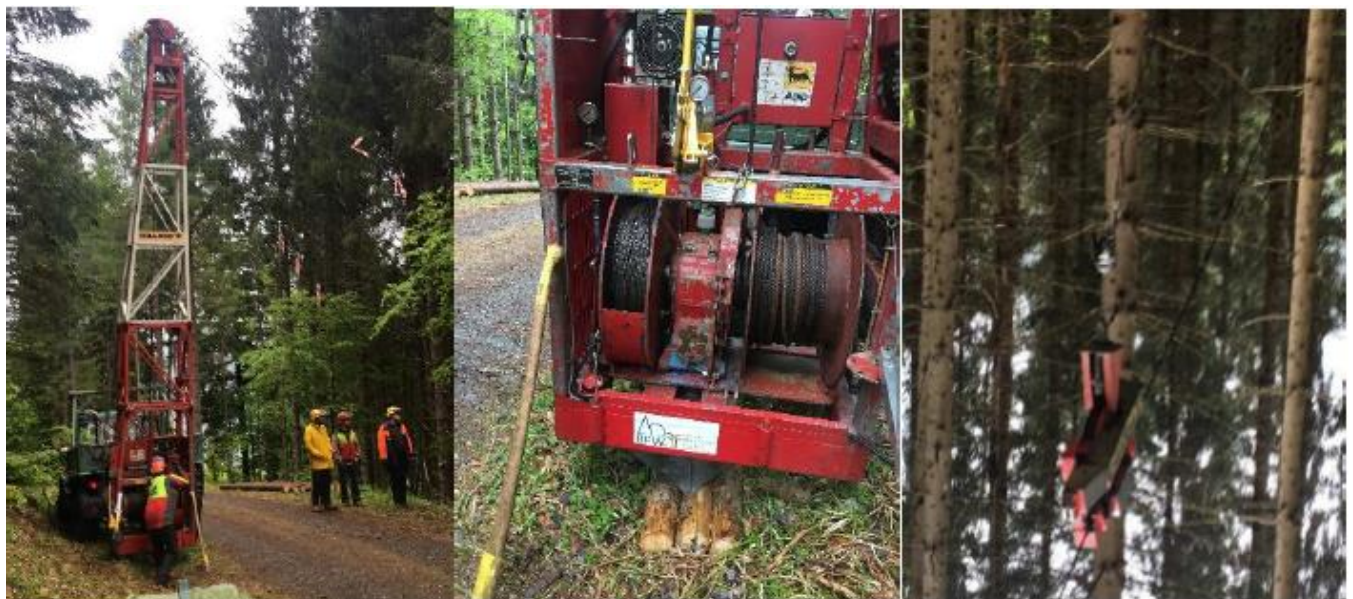
A medium-scale cable crane with tower and locking skyline carriage.
