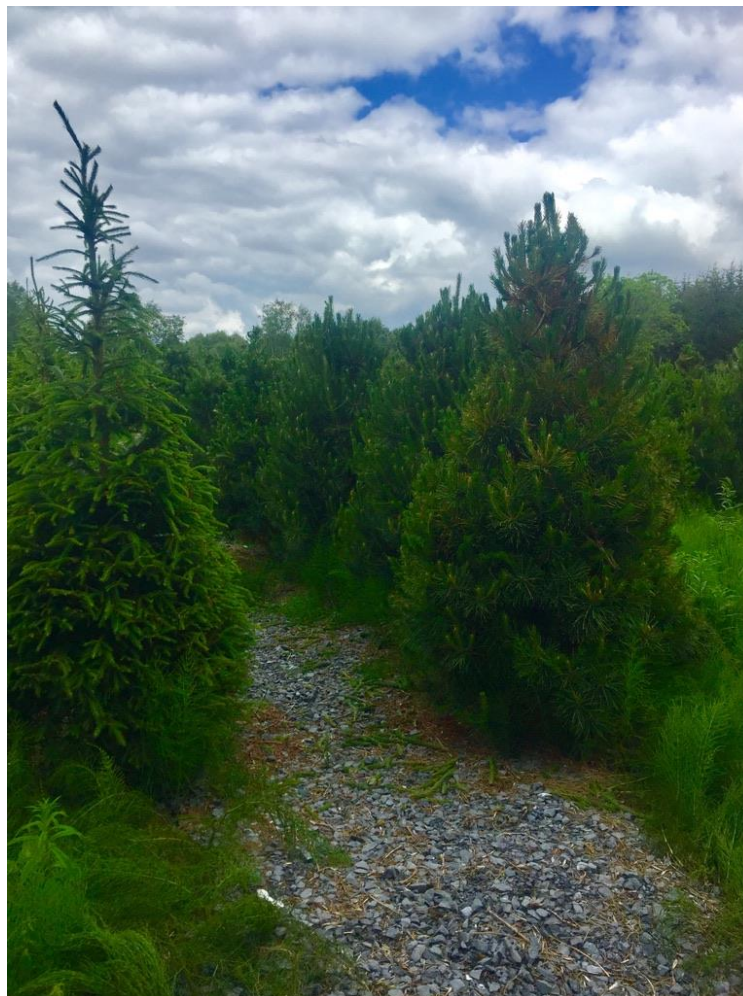
Path - drainage ditch filled to ground level.
