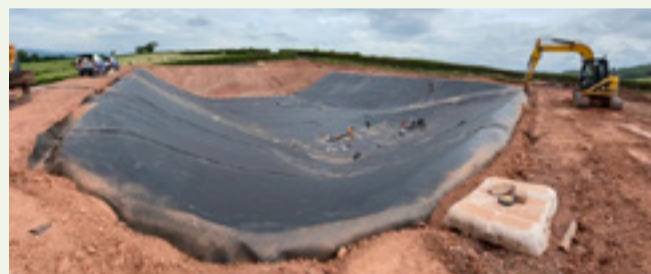
Figure 4. Slurry lagoon lining being installed at Graig Olway
