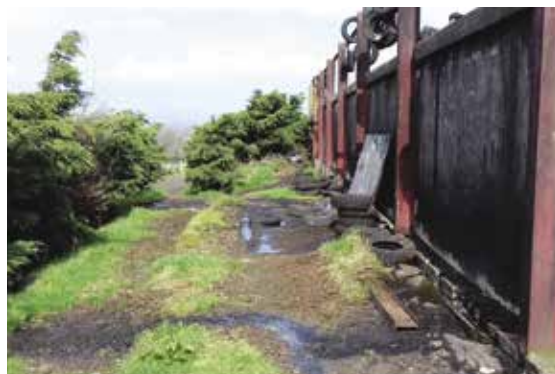
Example of a poorly maintained silage clamp without appropriate drainage, allowing effluent to leak, risking pollution to the environment.
