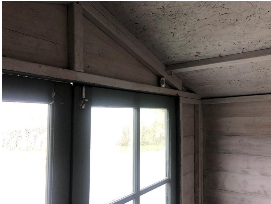
Passive Infra-Red Movement Sensor in Roadside “Honesty Box” Egg Shop
