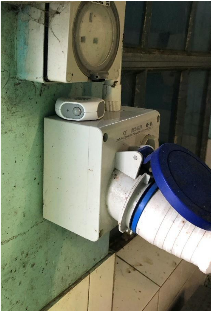
Passive Infra-Red Movement Sensor in Dairy and medicine store
