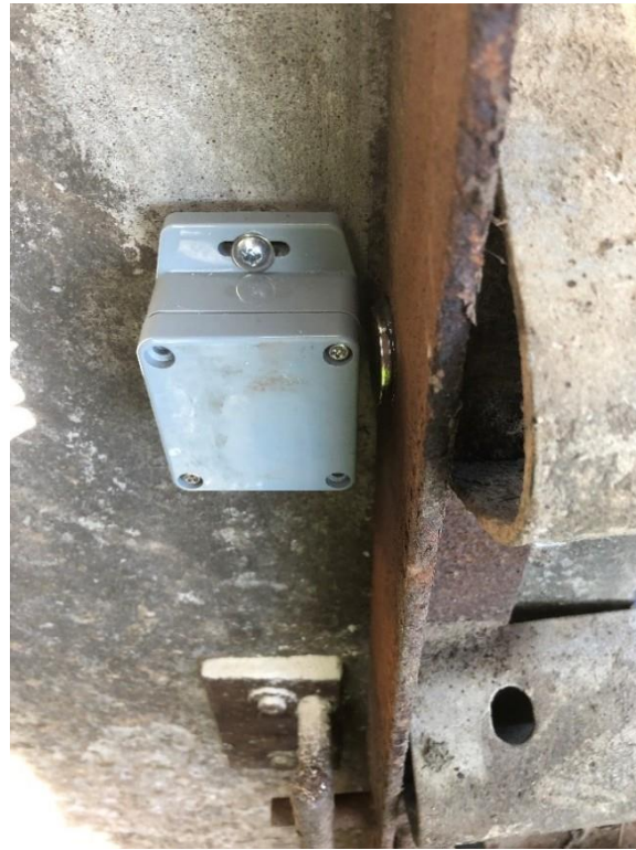
Open close sensor on gate post
