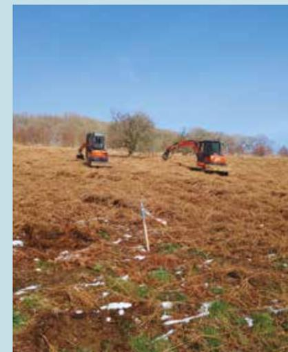
The mini diggers at work. One with a bucket and one with a rotovator attachment
