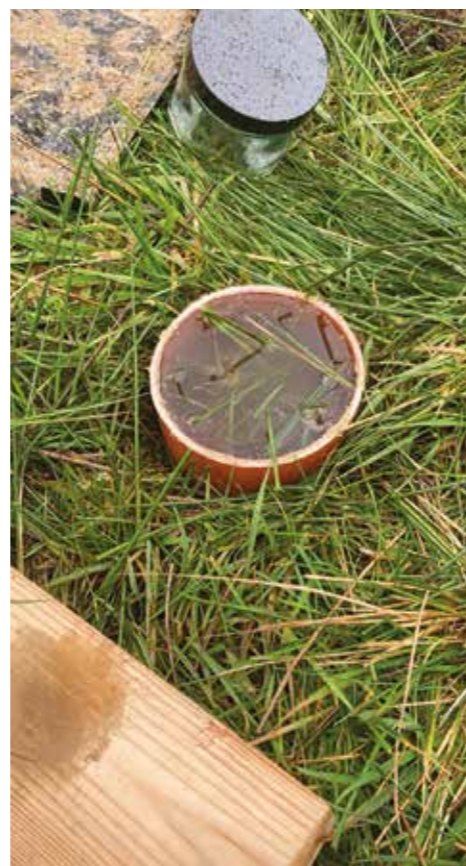
Water infiltration rates were extremely slow because the water could not penetrate the compacted zone.
