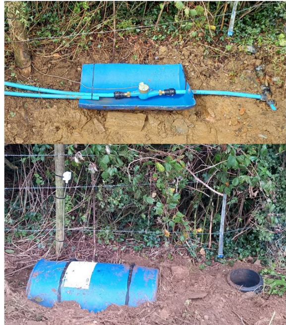
Figure 2. Site position installation
