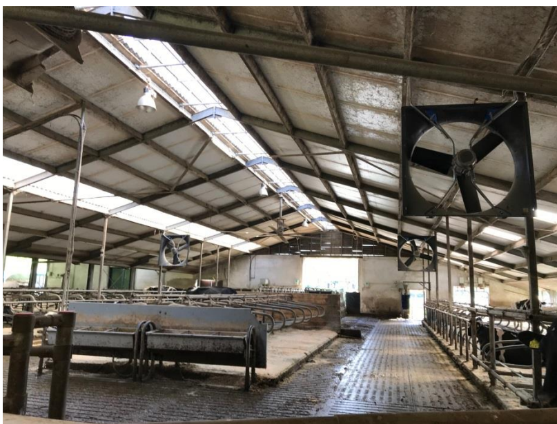
Note high ceilings, transparent areas of roof, fans, making the shed light and airy. Most cows were outside grazing when this picture was taken.
