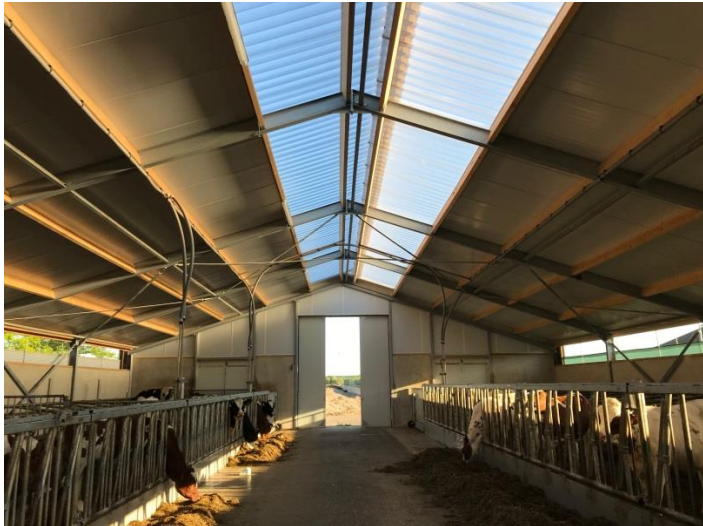
New shed built last year for young stock. Note transparent roof and automated shutters.
