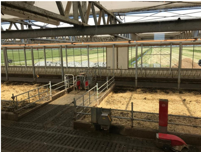
Deep litter housing with slats. Open sides with automated shutters, transparent ceiling and scraper robot.
