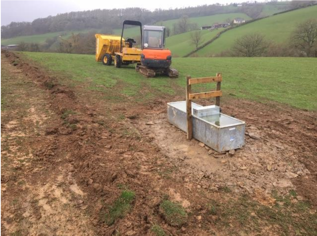
Installing the water infrastructure at home. Spring 2019.
