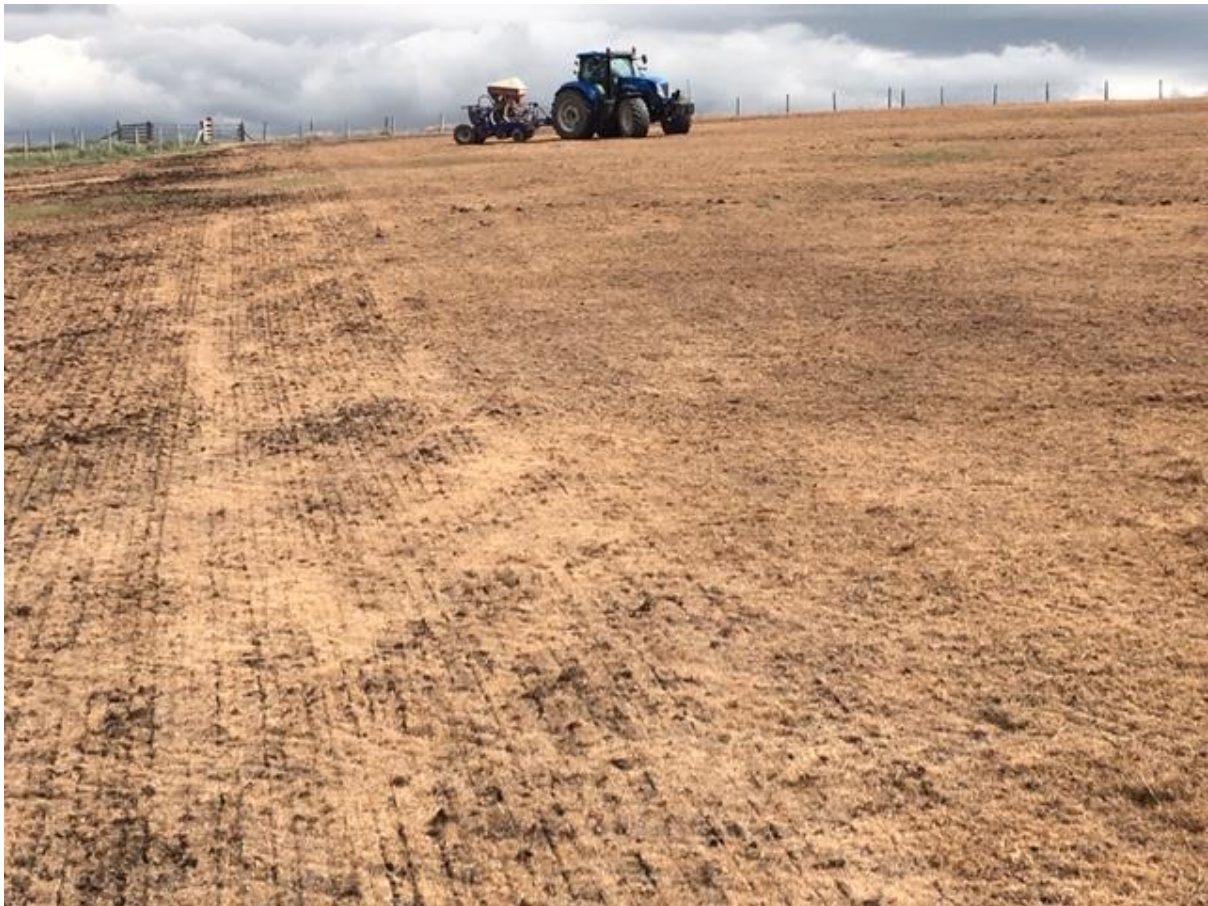
Showing surface after seeding with a Moeres Unidrill on the left of the photo, two passes of the OPICO Harrow on the right.
