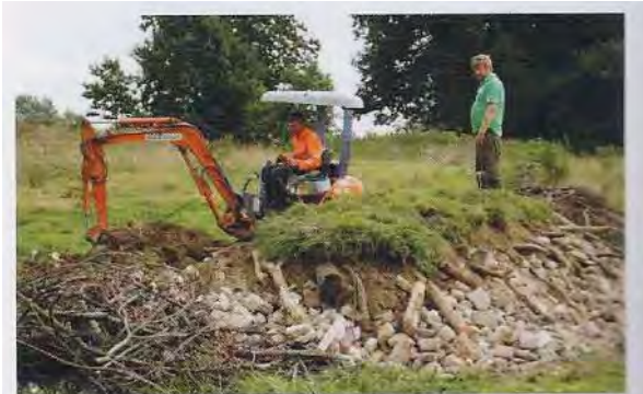
A reptile bank under construction. Turf has been stripped to create a shallow pit to receive a pile of hardcore and logs. This will be covered with the stripped turves (Lee Brady)
