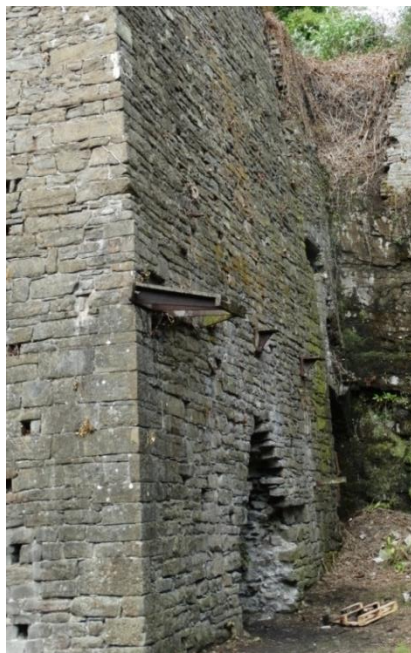
Illustration One and Two showing the precarious structure of Furnace No.1.
