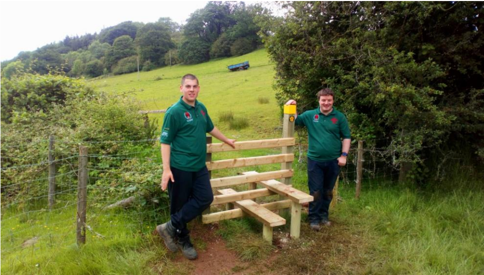
Installing Rights of Way, footpath diversion stile – June 2019
