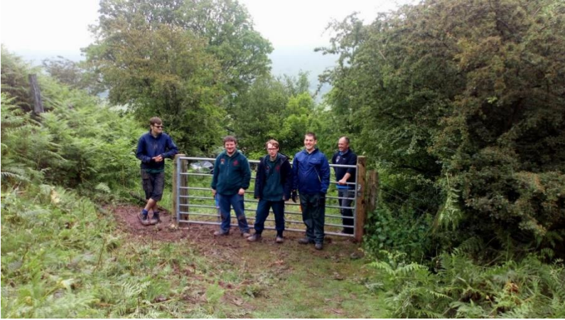
Gate Installation and Vegetation clearance, Cwmyoy - June 2019
