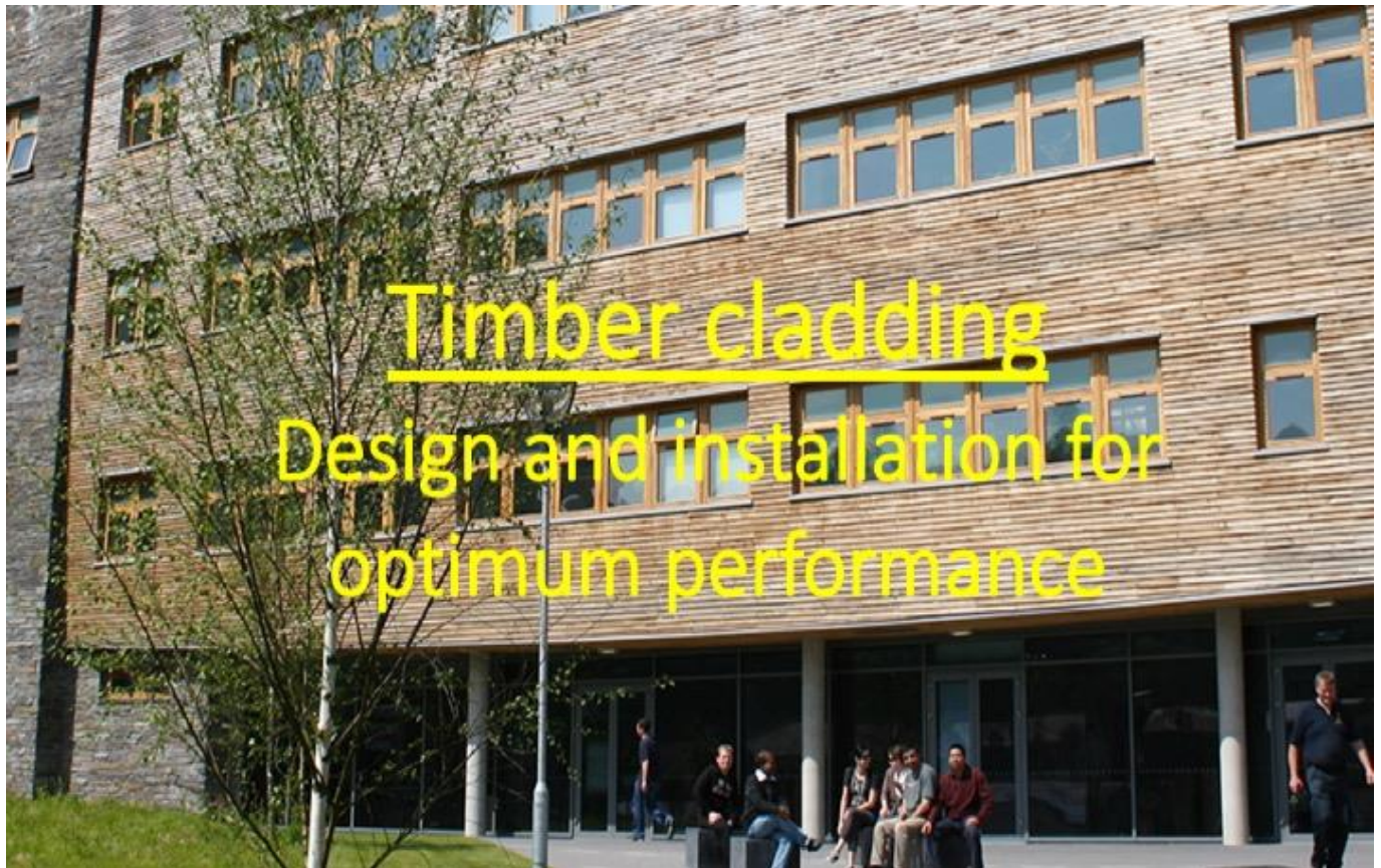
Environment Centre Wales Building, Bangor
