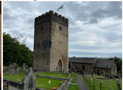
Church, tower and grounds
