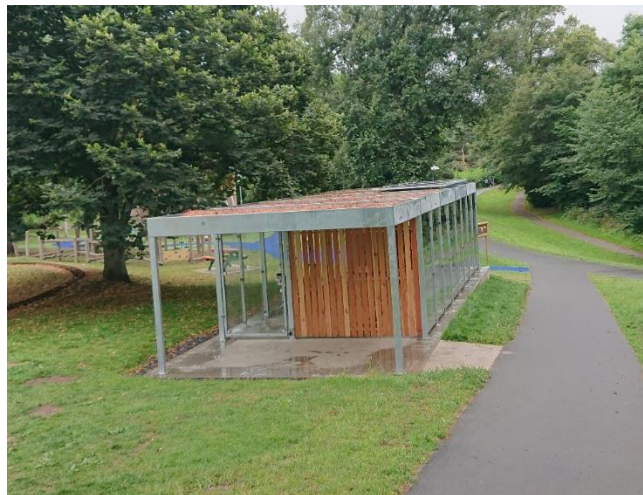
PV panels mounted flat on the roof of the bike hub, providing light and charging for electric bikes.
