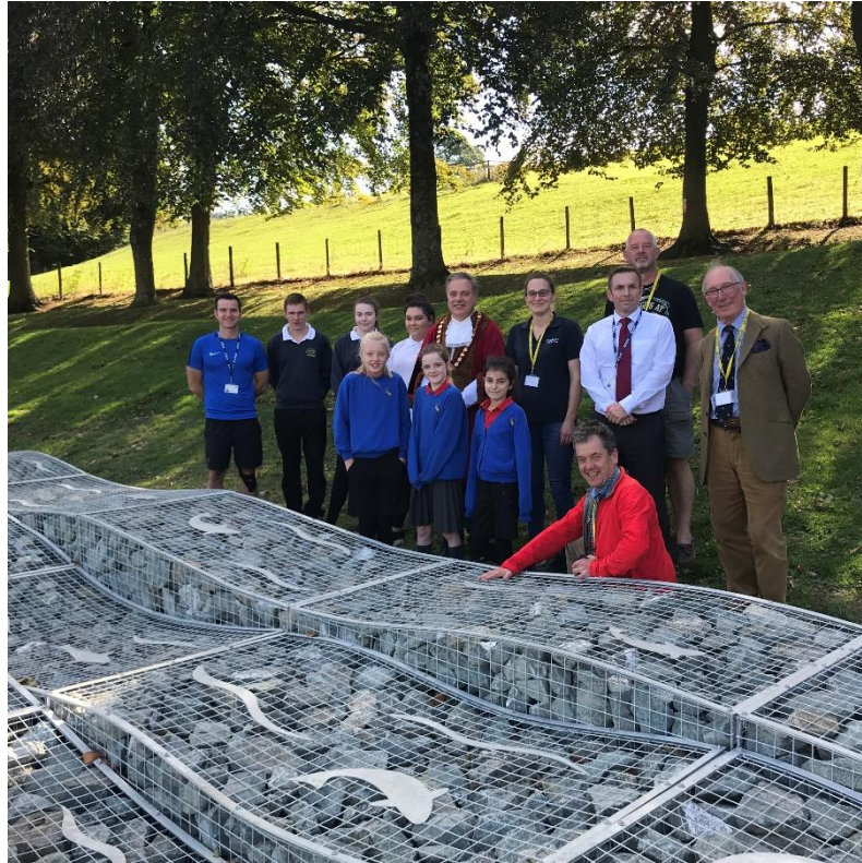
Photo showing the Llanfyllin High School rain garden, opened with transition activity with Llanfyllin Primary School
