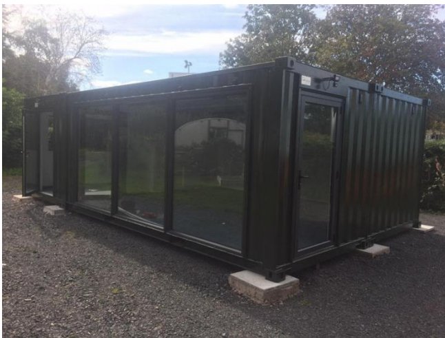
2 shipping container training rooms
