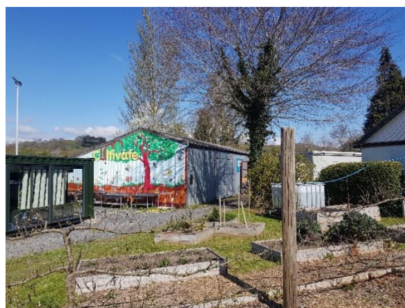
36. Old shed which accommodates Bikettf and the Community Shed Project
