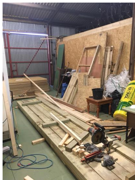
15 Assembling the materials for construction of the community space project
