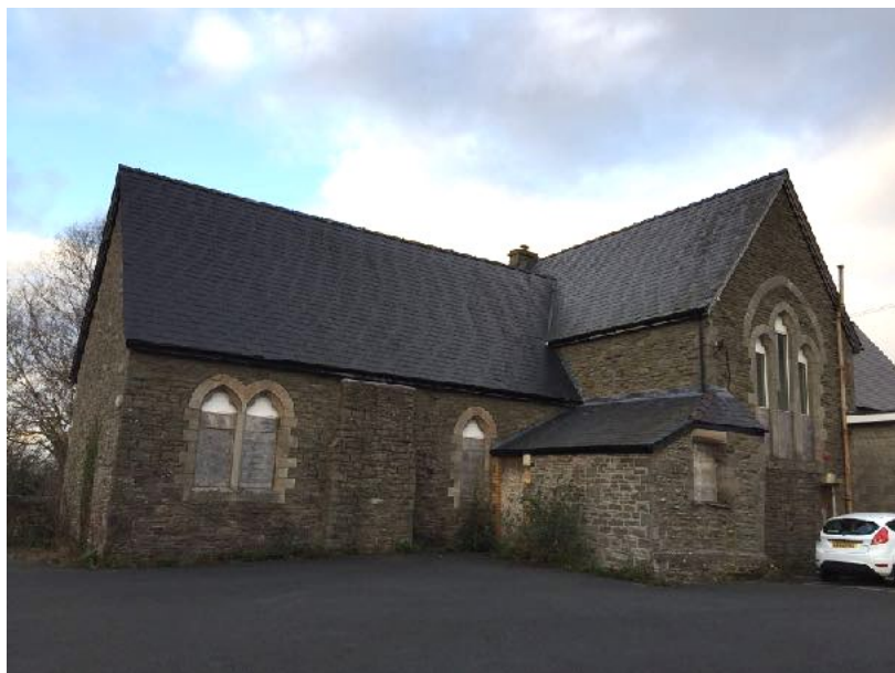
Southern frontage, lower section.
