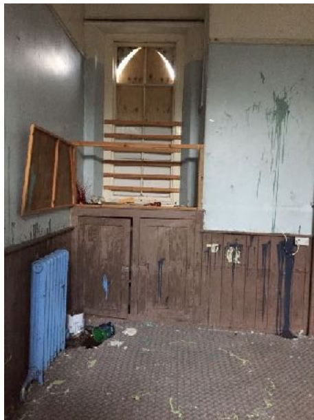
High windows in central section
