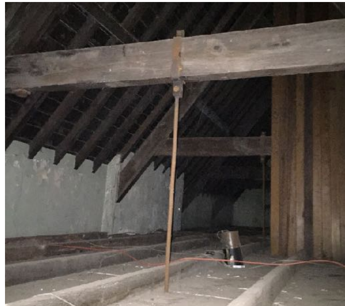
Attic space over top, eastern section.
