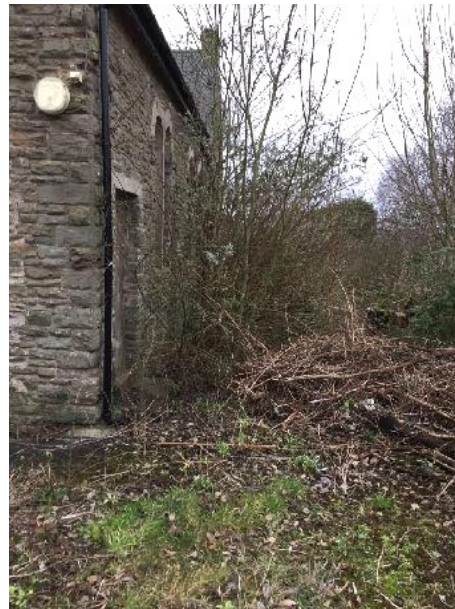
Vegetation along rear elevation,
