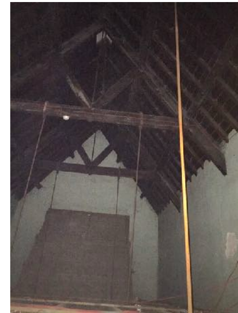
Attic space over central section.
