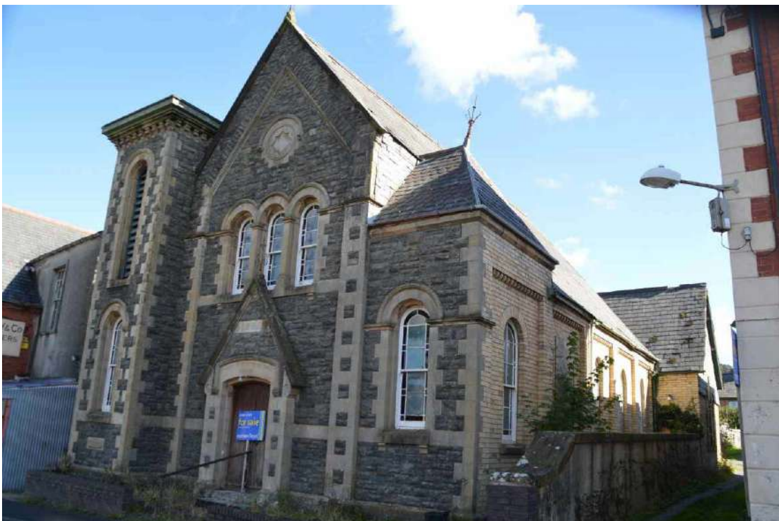
Plate 2: Bethel Chapel (school room to rear), looking north-east
