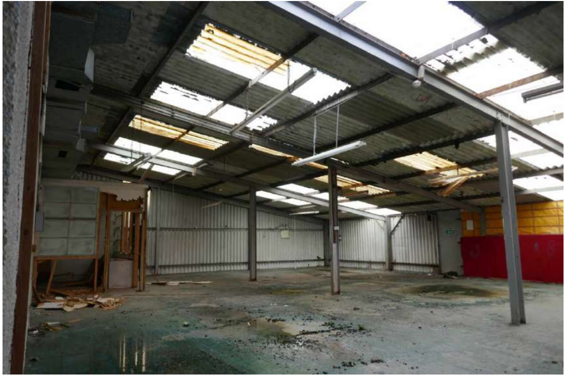
Plate 13: 1970s extension to rear of Hall, before renovation, looking north-west
