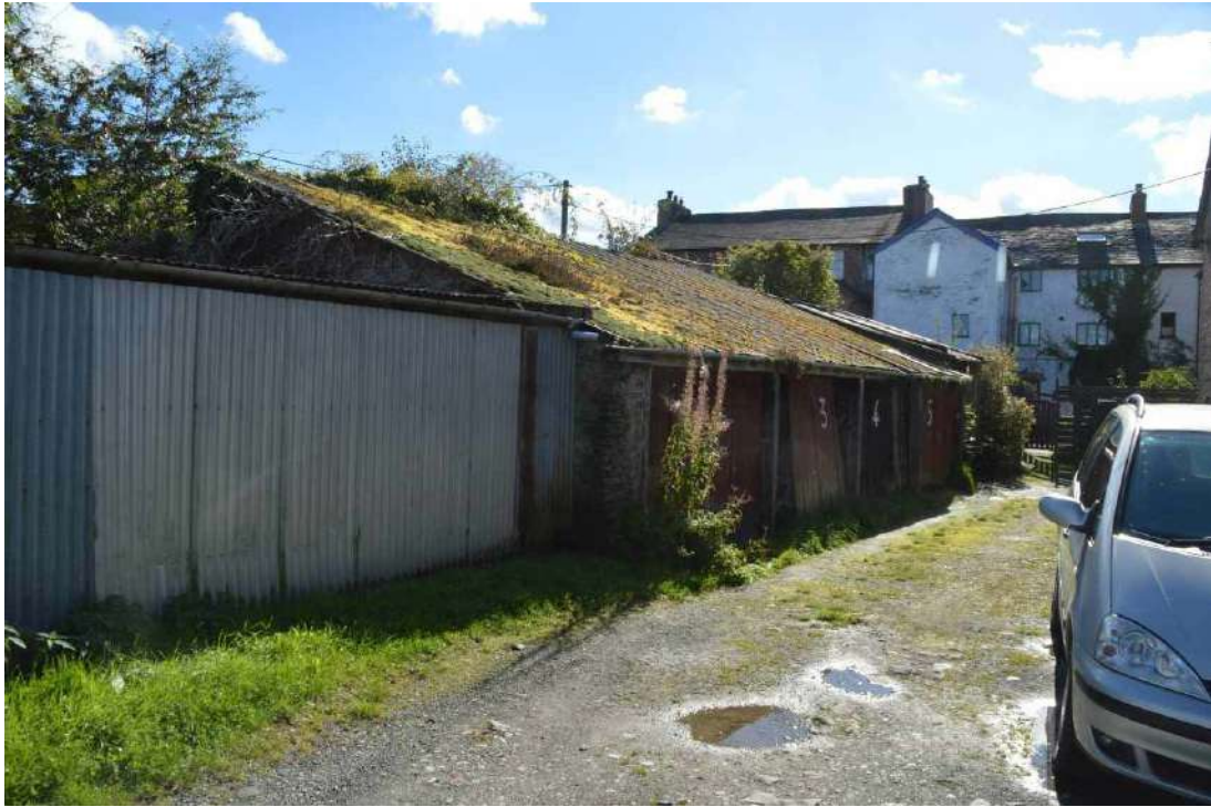
Plate 15: Garages, looking south
