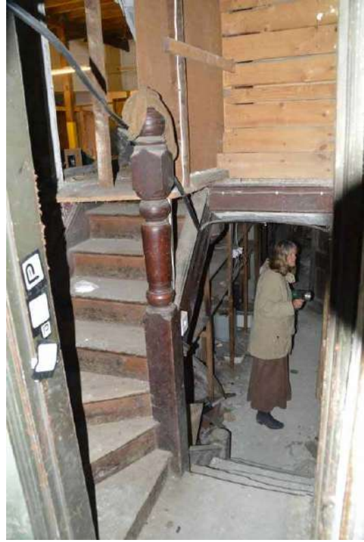
Plate 10: Steps between basement and stage
