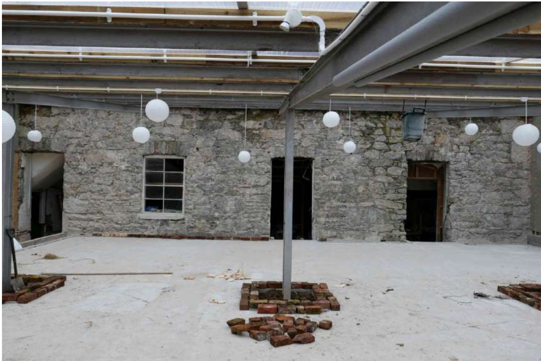
Plate 13: Rear, stone wall of Hall during renovation work, looking west
