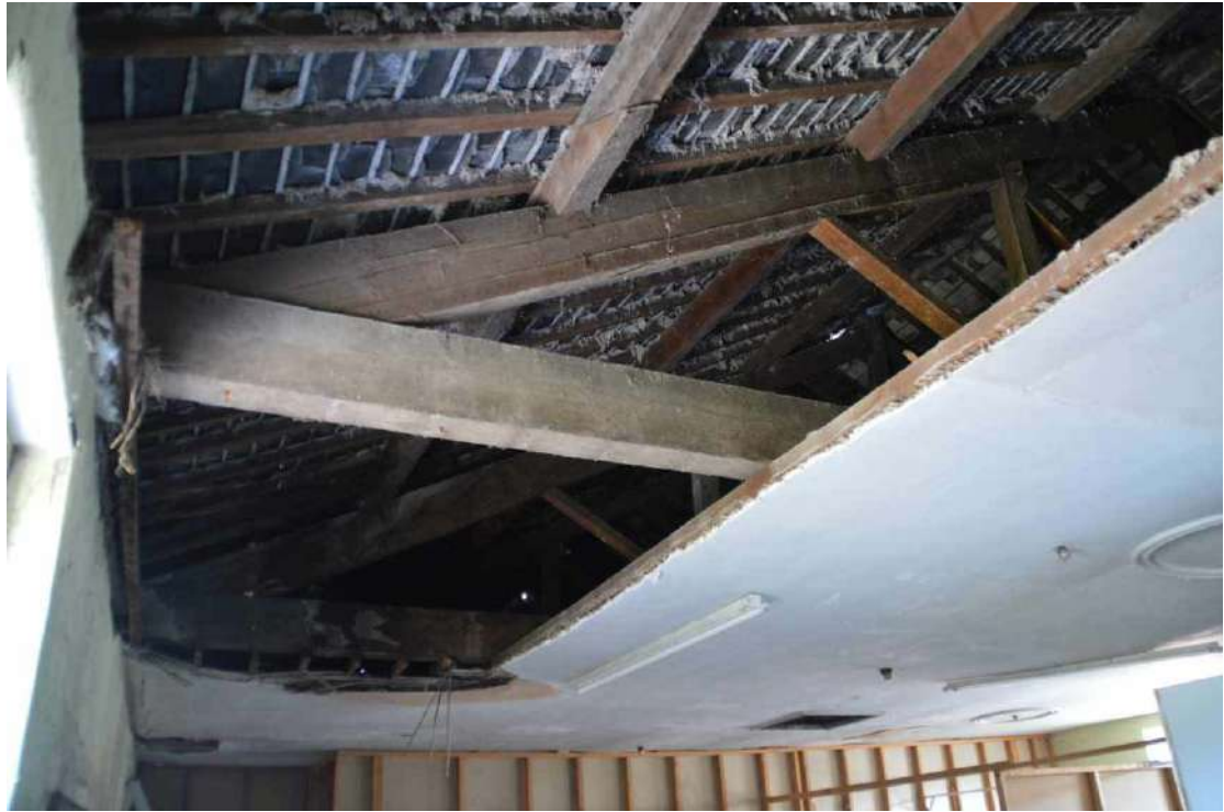
Plate 12: Timber frame in upstairs of Hall, looking north
