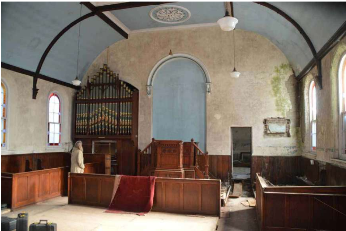
Plate 4: Interior of Chapel, looking east
