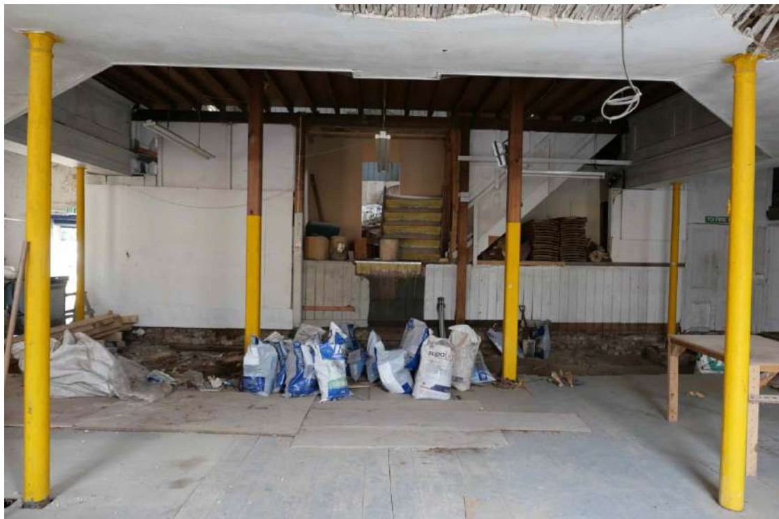
Plate 8: Interior of Hall showing stage area, looking west
