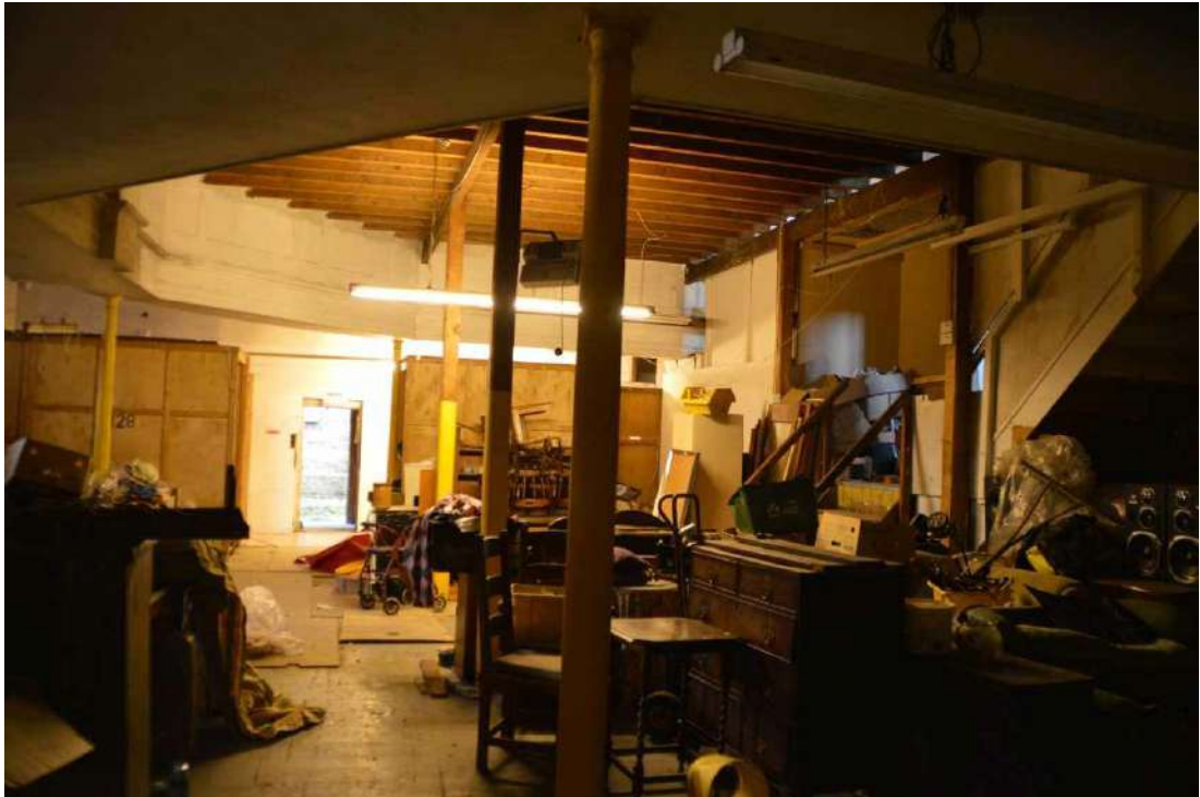
Plate 7: Interior of Hall with floored over void, looking south
