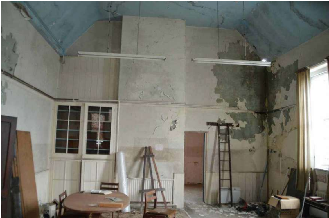
Plate 5: Interior of School Room, looking north
