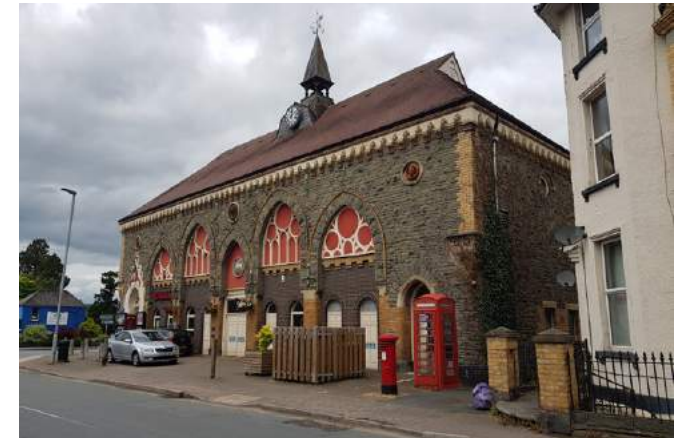
South main elevation of WAC as seen from Castle Street
