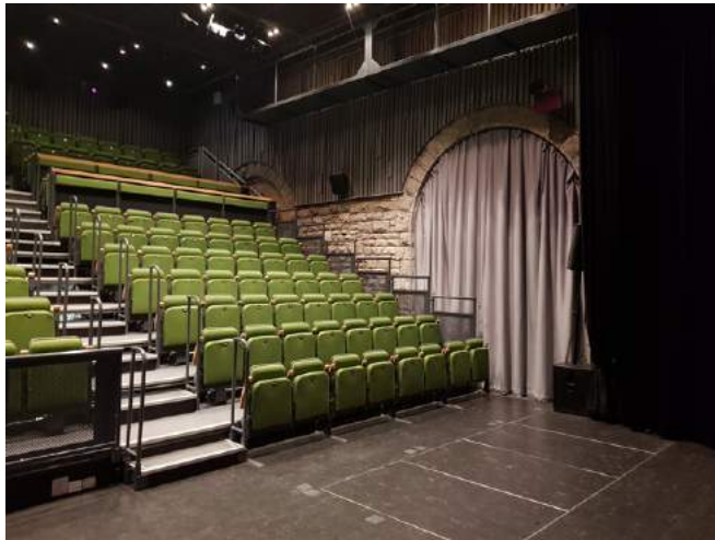
Market Theatre - 2012 Retractable seating and acoustic panelling to be maintained
