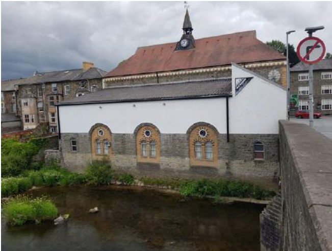
View from the Bridge over the River Wye : an important convergence of all traffic from both the A470 & A483 through the middle of Wales
