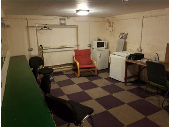
xR.1.06 - Slab broken out to become stage level Accessible Dressing Room
