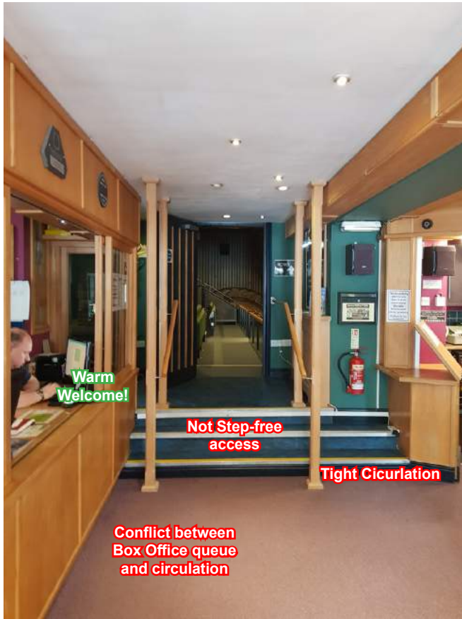
Existing Box Office & Balcony Access
