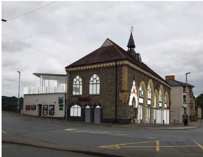
COLLAGE - South West approach from Castle Street
