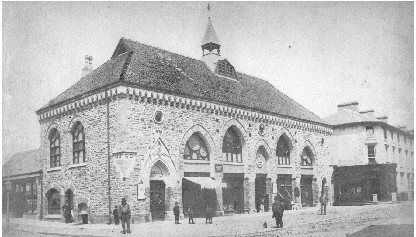
Early days - mostly likely 1880's as there is no clock installed yet.
