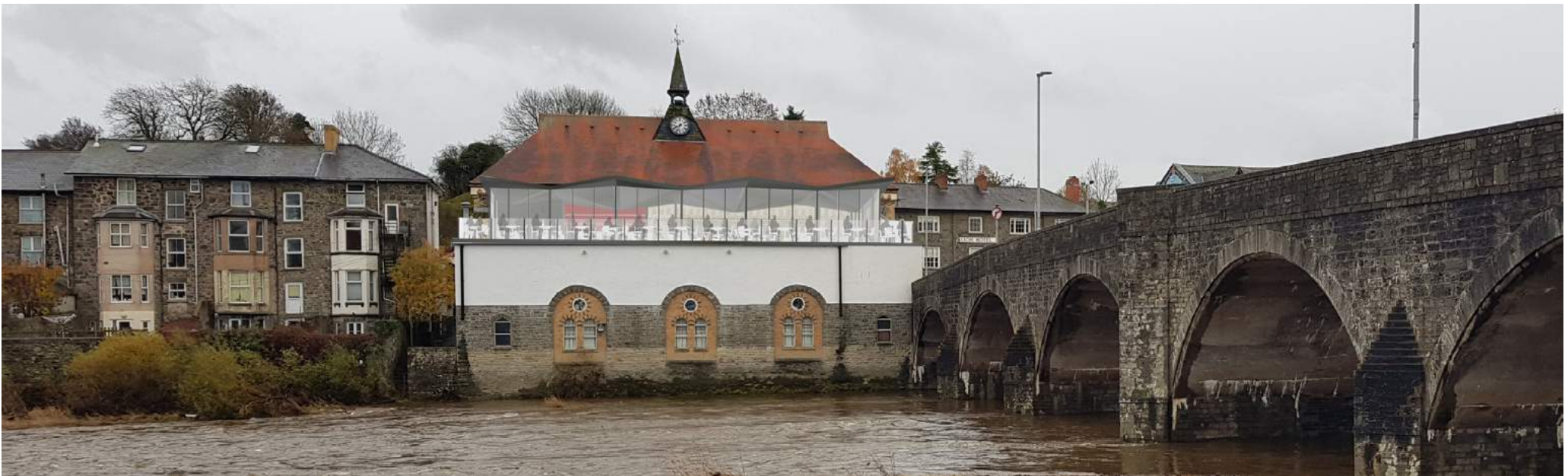
Collage view from the northern bank of the River Wye
