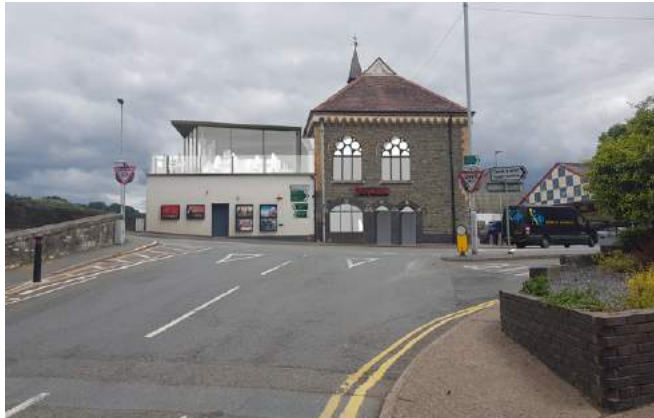
The natural tendency is to want to head straight towards the building but the reality of crossing by the bridge is dangerous for pedestrians, especially the young and the elderly.
