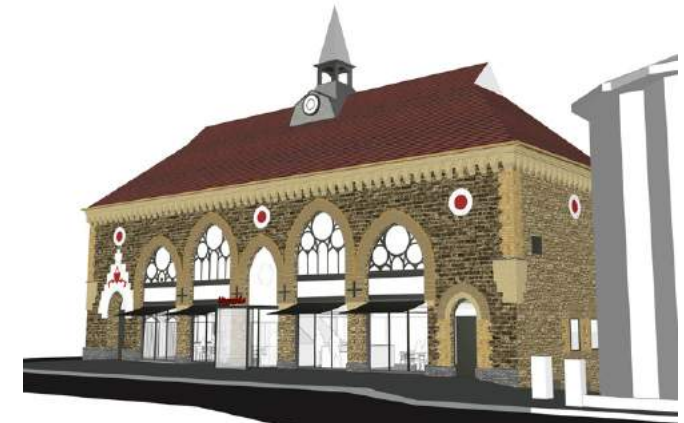
3D study of elevation with central glazed porch that projects beyond the line of the masonry building in the same way the previous cast iron canopies once did.
