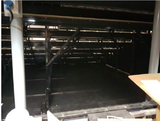
The space under the rake needs to be kept clear but we can build in front of the columns.
