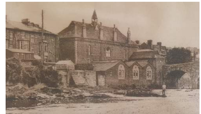
Early photograph of the Market Hall within its three gables
