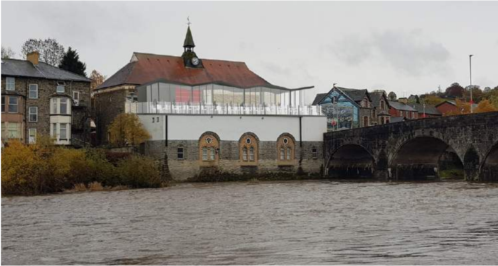
Collage view from the northern bank of the River Wye
