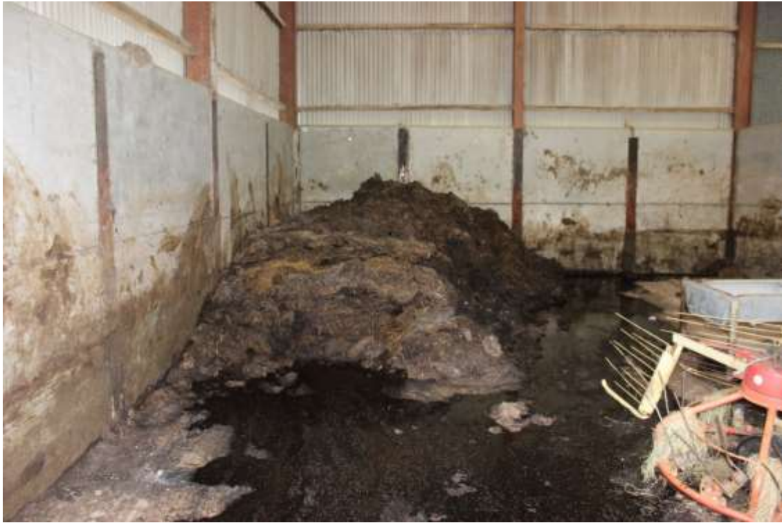
Plate 5 – Dolobran, internal storage of manure on hardstanding. Liquid is collected via slot drain.
