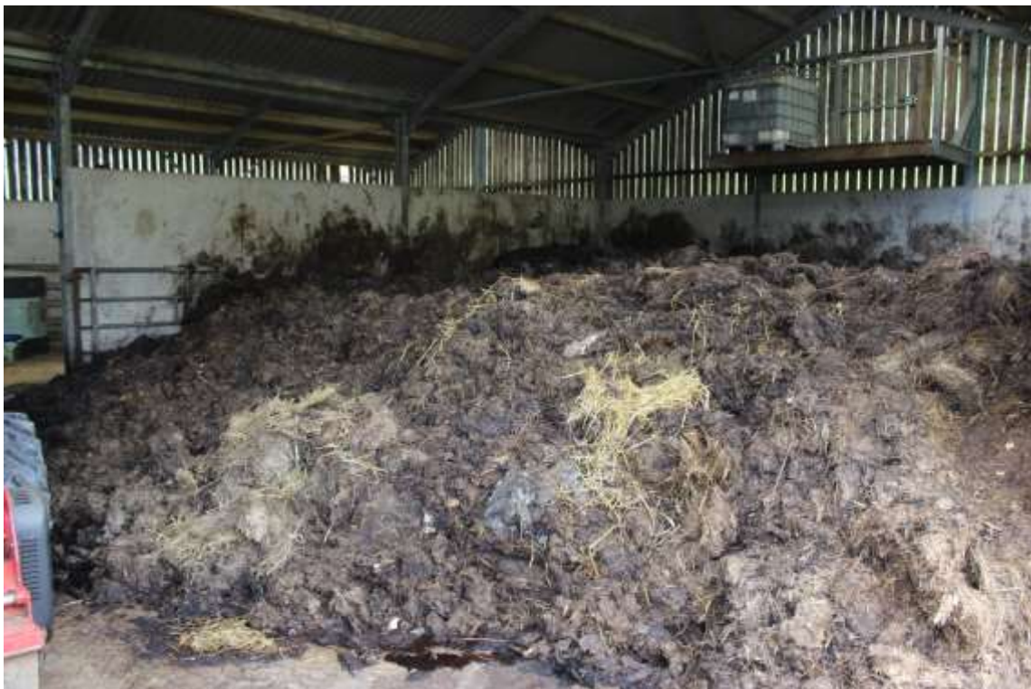
Plate 12 – Hafod y Llan, internal storage of manure. Liquid collected via slot drain
