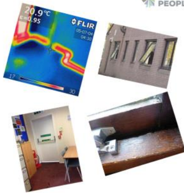
Here you can see some of the issues relating to insulation. Top left: Heat being lost from un-insulated pipes Top right: Windows being opened whilst the heating is on Bottom left: Example of a draughty door Bottom right: Example of a draughty window
