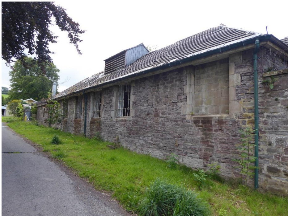
Fig 7 Single storey Workshop block to east of Main Block
