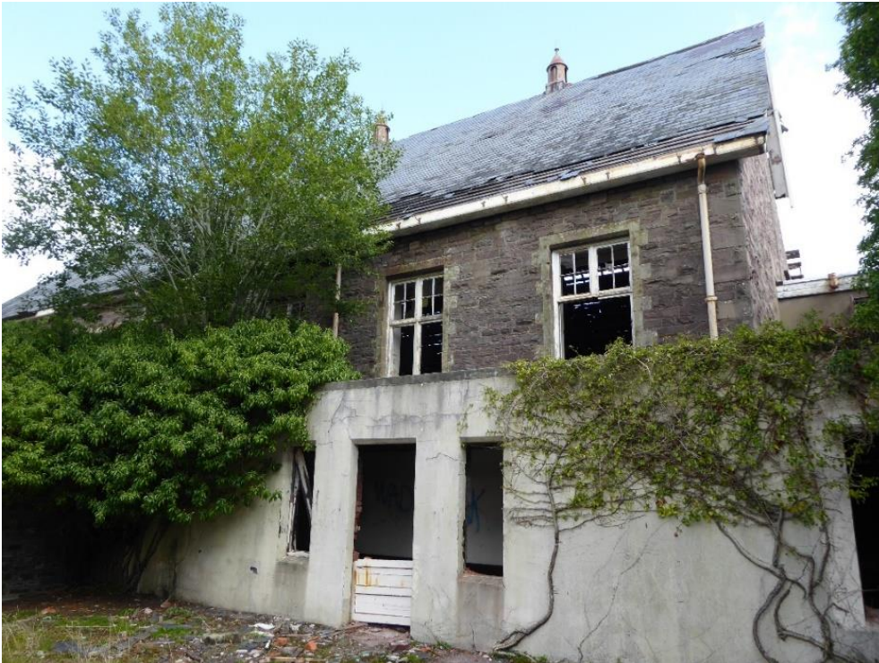
Fig 13 Former Dining Hall to centre of the hospital complex
