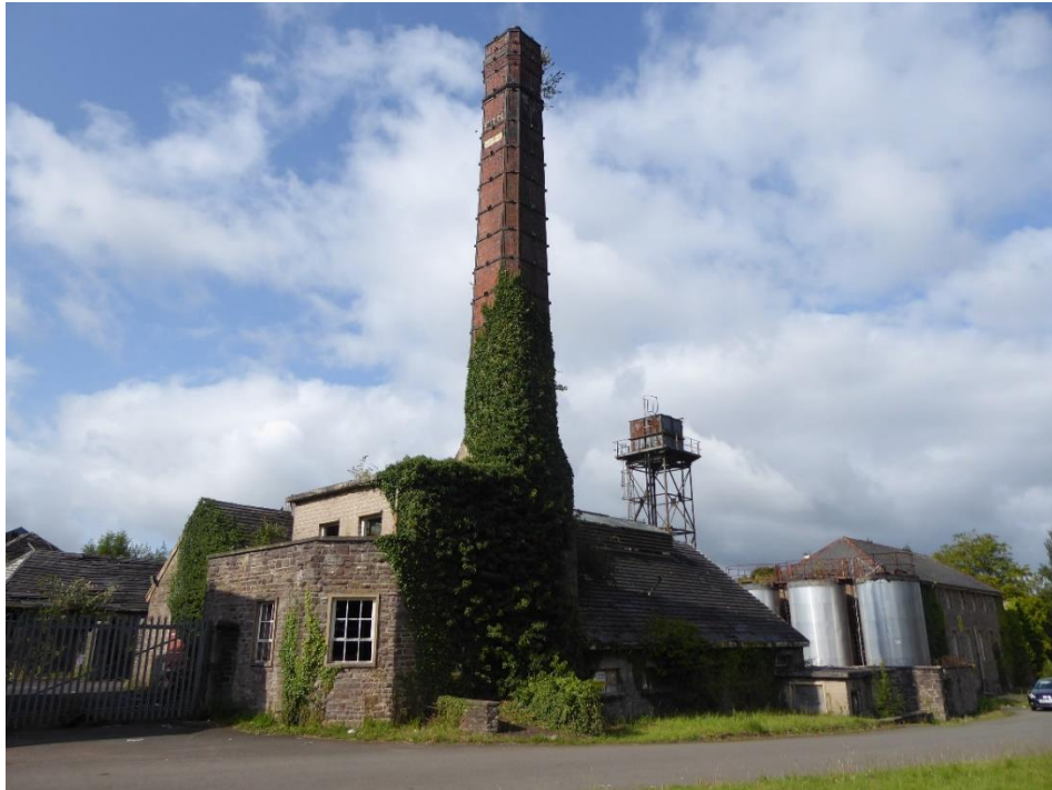
Fig 5 Chimney to former boiler house, to west of main (official) block
