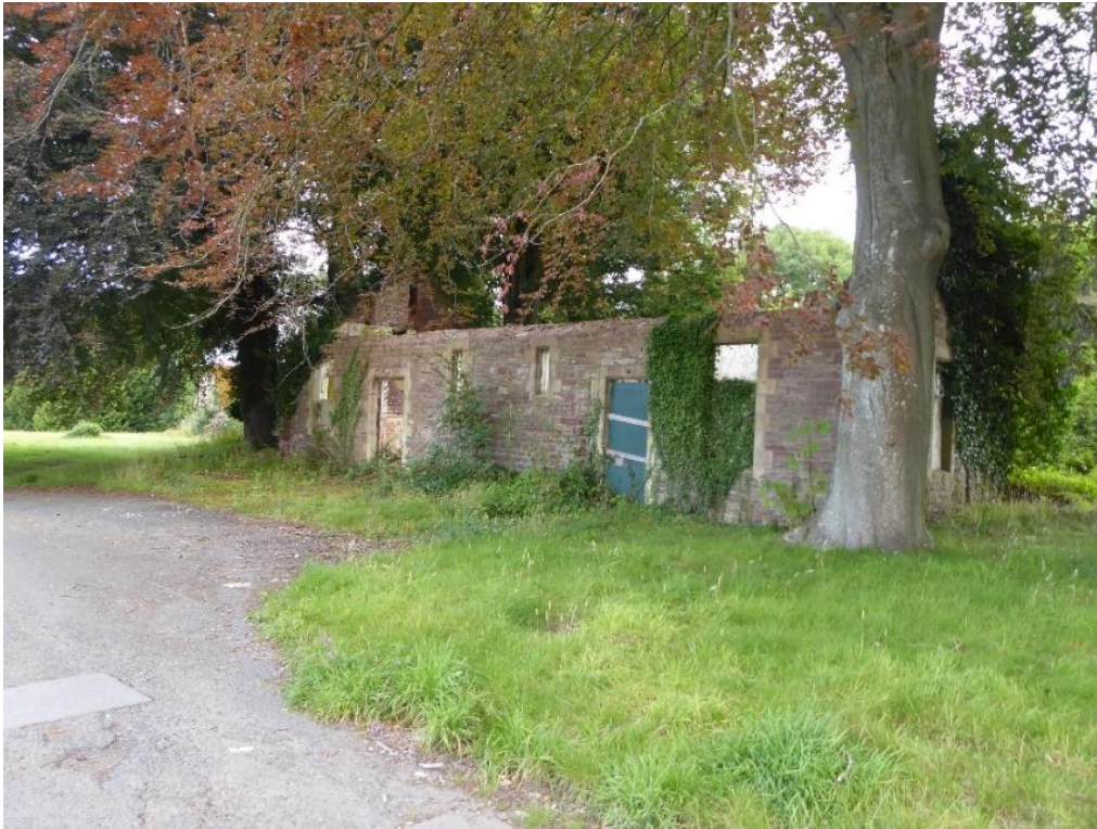
Fig 10 Former Mortuary to south east of chapel
