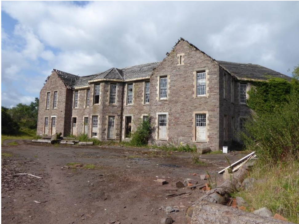
Fig 11 2-storey range to south-east of original hospital complex
