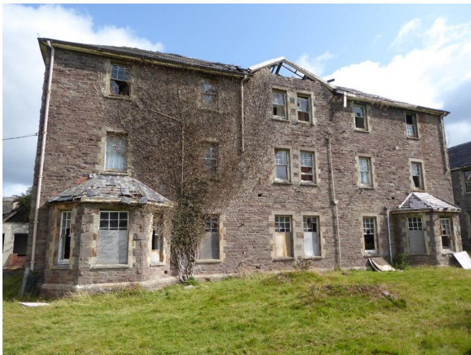
Fig 12 3-storey block to south side
