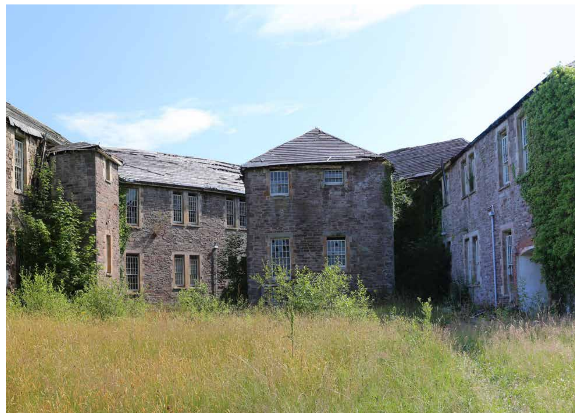
Existing courtyard and buildings within Former Mid Wales Hospital Site
