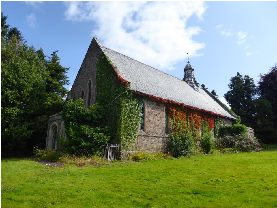
Fig 8 Chapel viewed from south-west
