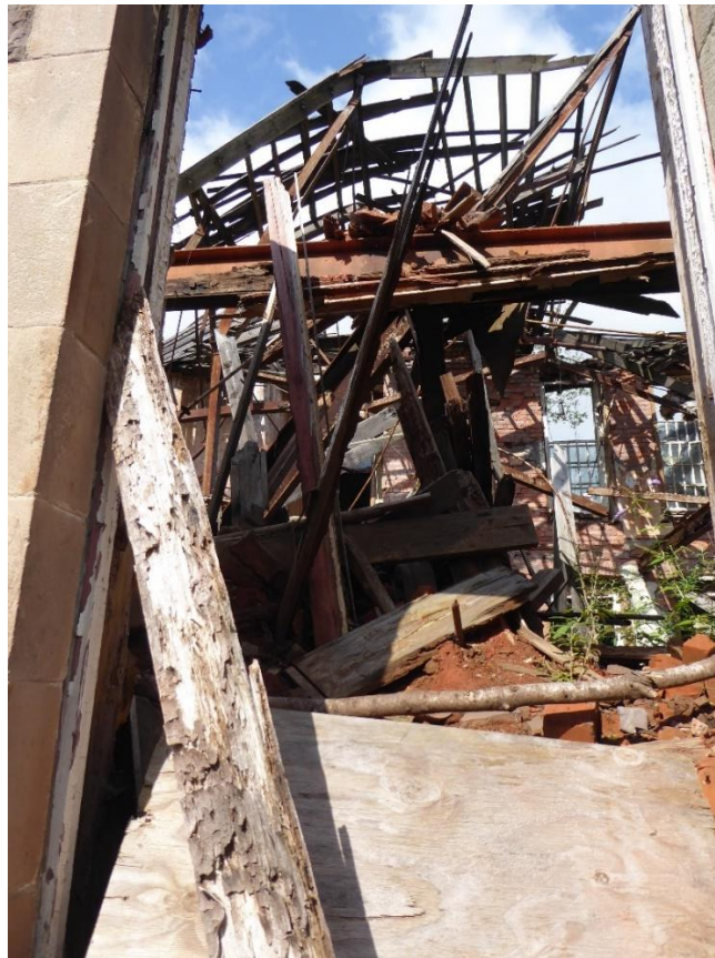
Fig 15 View into block to south-east of site
